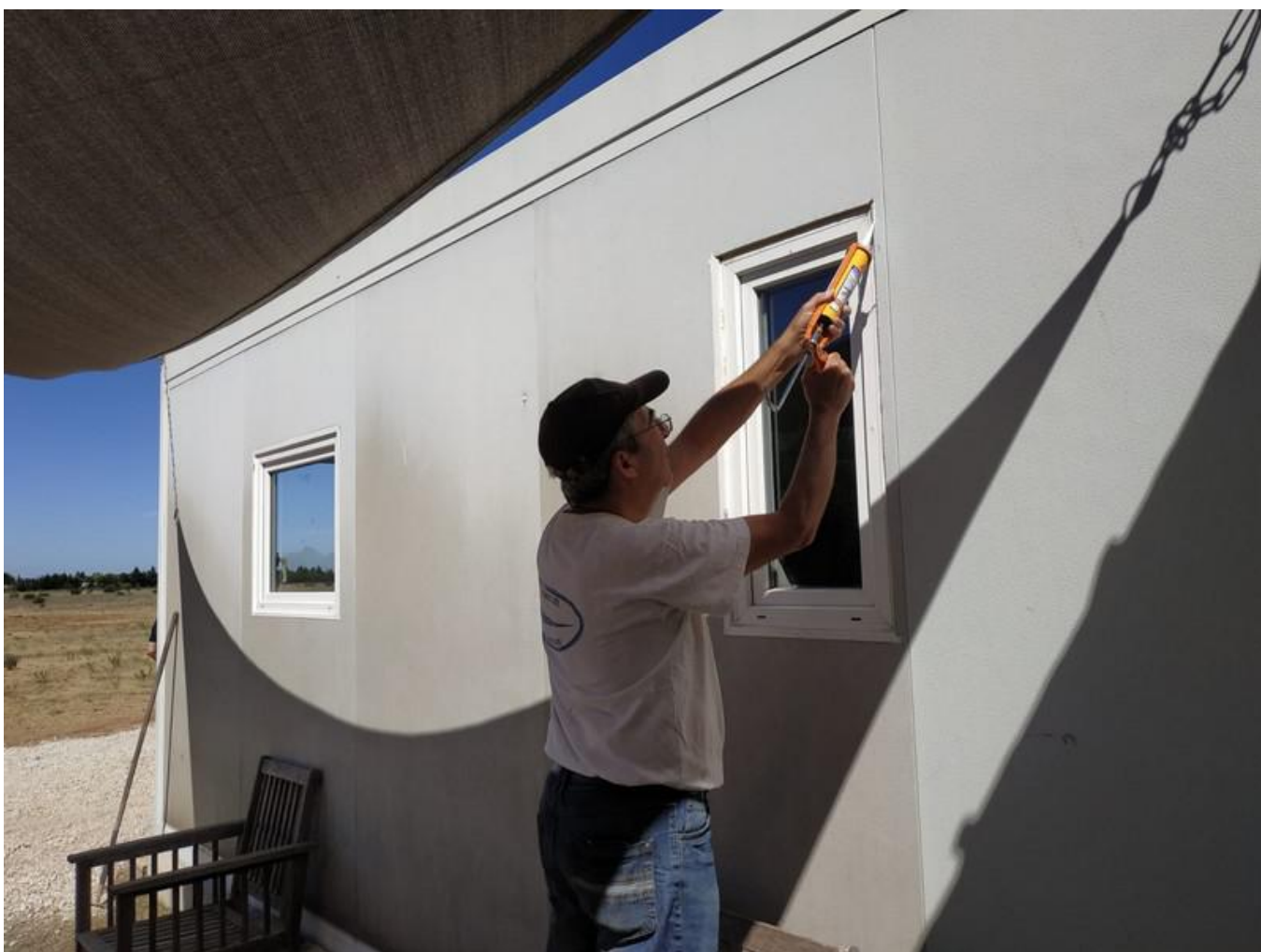
Finition des joints.
